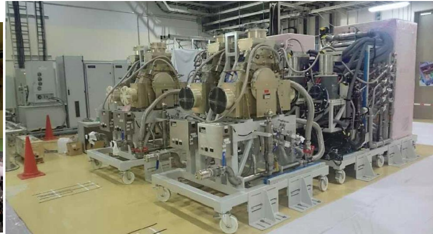
RF system partially installed at Rokkasho
