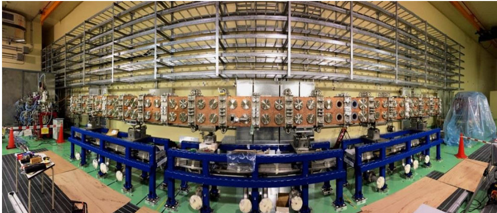
RFQ recently installed at Rokkasho
